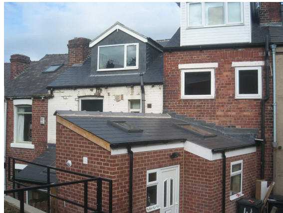
Photograph 2 Extension viewed from the rear garden of No. 27
