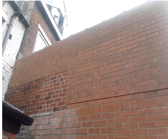
Photograph 1 Extension viewed from the rear yard of No31.
